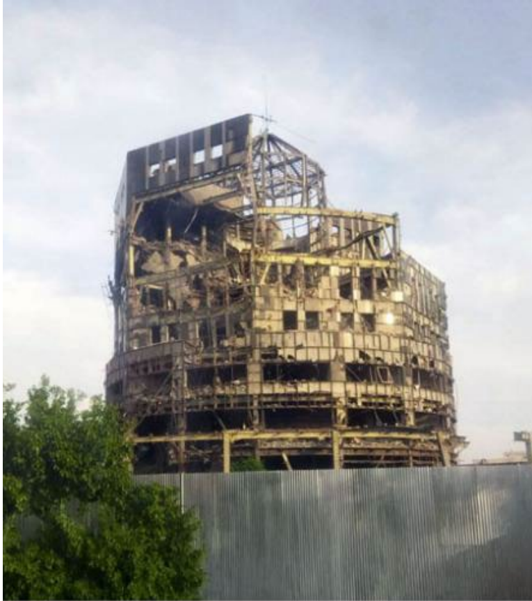
Extensive destruction of the Iran Space Research Center following airstrikes ©HRA
