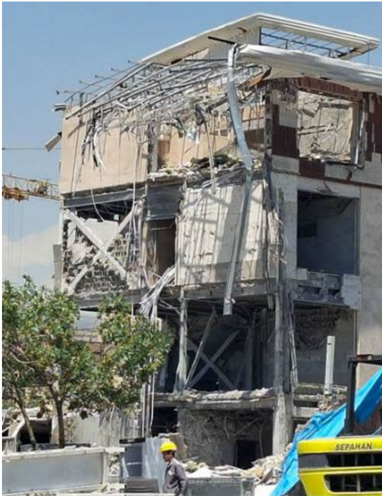
An administrative building that was subjected to repeated strikes ©HRA
